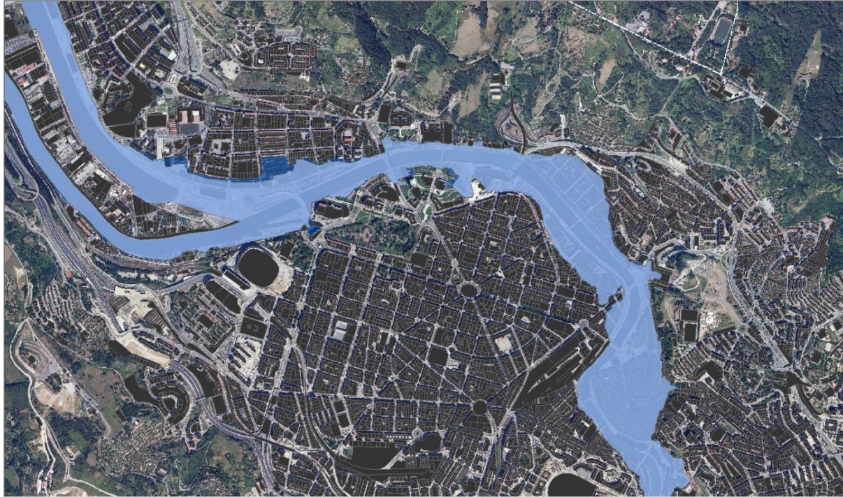
Figure 3. The 500-year return period flood risk map. In dark blue the areas affected without the opening of the canal, while the light blue area represents the potentially flooded areas once the canal has been built.
